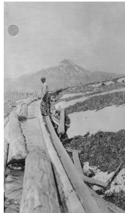
Log flume which conveyed logs from Mount Haggin over the Continental Divide and into the Clark Fork Valley
