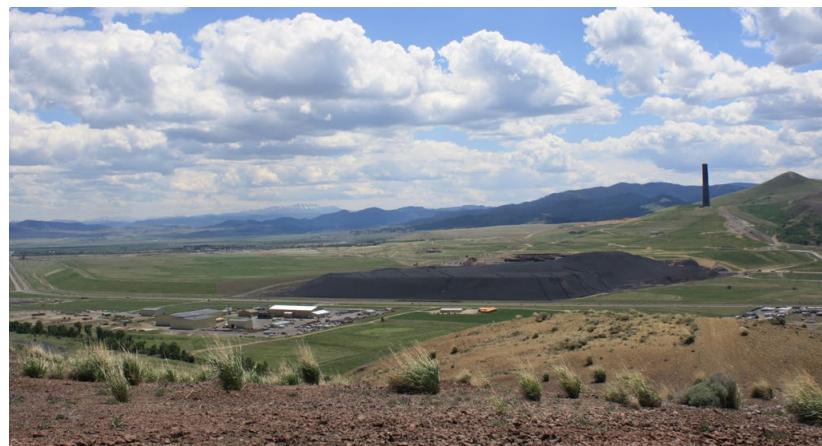
A view of remaining slag near Smelter Hill. The green hills surrounding the black piles have been remediated with cap and cover system.
