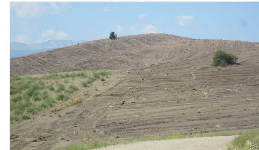
Stucky Ridge after grading. Photo NRPD.
